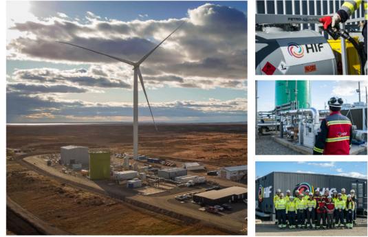
Location: Tehuel Aike Estate, Punta Arenas, Magallanes Region, Chile
